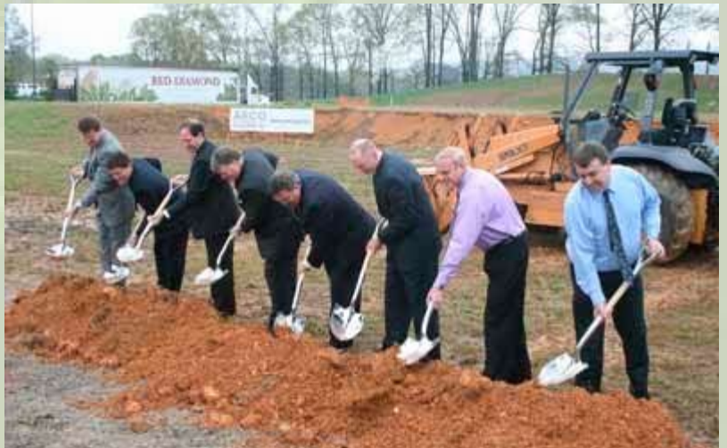
Red Diamond president Bill Bowron, center, and other officials break ground on a food-service distribution center at the corporate campus in Moody.
